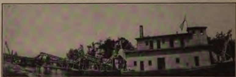
Ladder Dredge operating on Fox River, Wisconsin. Figure 99.
